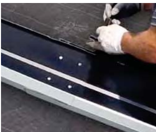
Install inner gable as a whole piece. When adding a second inner gable trim, open up the water lock and cut out the top section to allow for tight, overlapping, waterproof fit.
