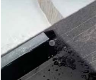
Cut bottom of inner gable so outside weeping channel will protrude past drip edge ¼".
